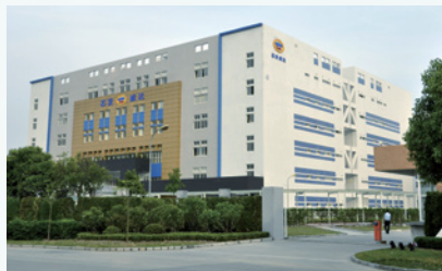
Armolink Site in Shanghai, China
